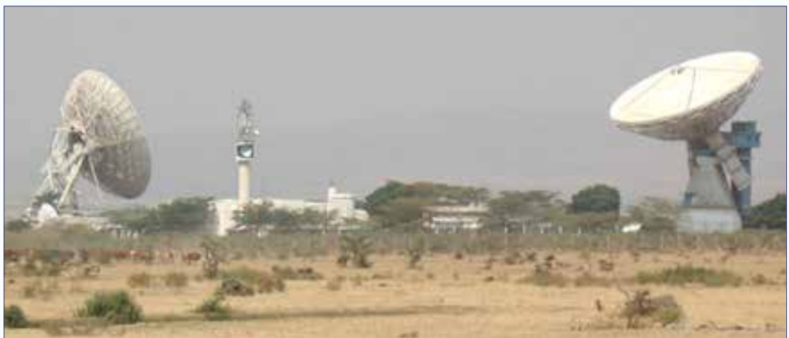
Longonot Earth Station
